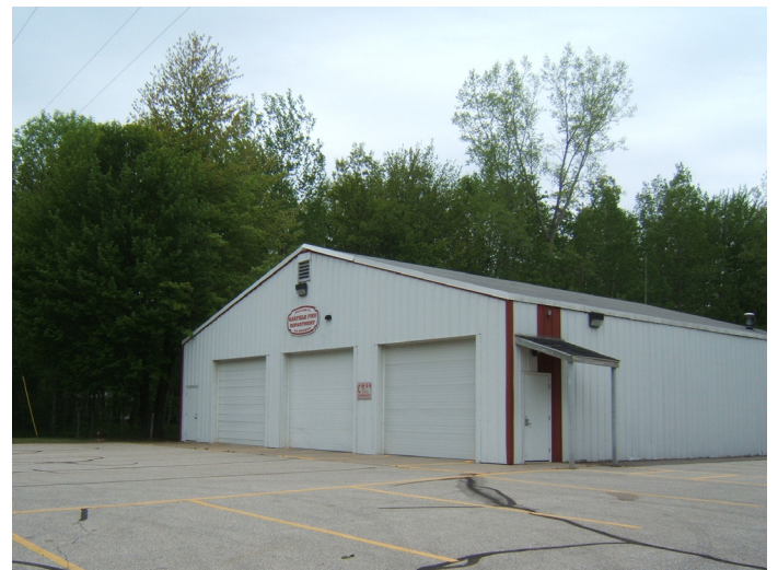
Garfield Fire Department Station No. 1
